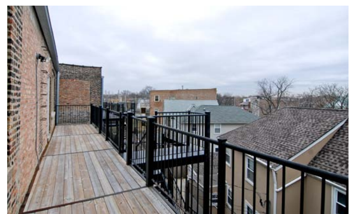
Oversized open deck overlooking single family homes
